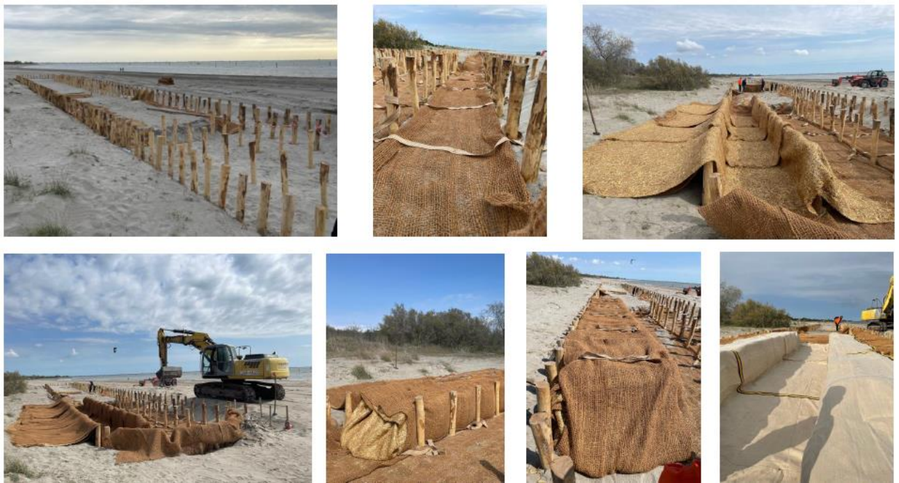
Figure 8: Initial phases of the artificial dune construction
