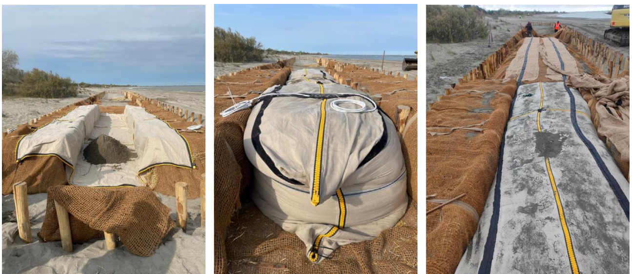
Figure 9: Coir bag technology within the artificial sand dune
